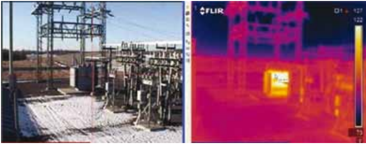
Digital photo and IR image of a substation showing a transformer with excessive temperature.
